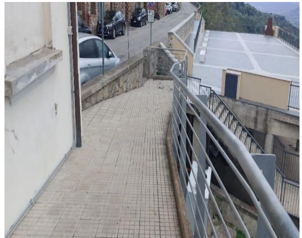
46 Common entrance ramp
