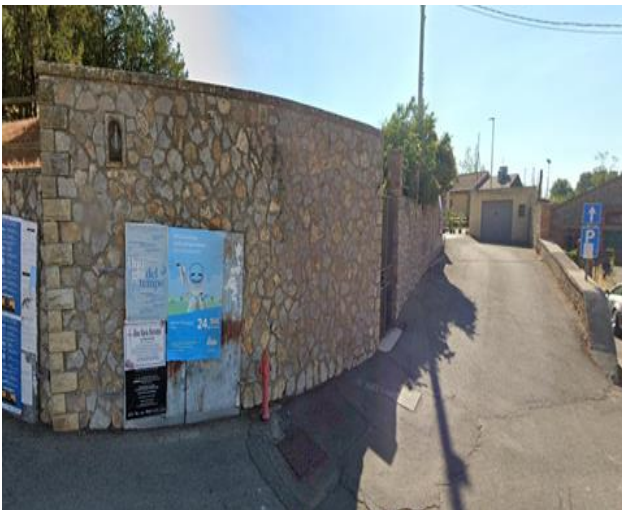
6 entrance to the Poggionovo car park
