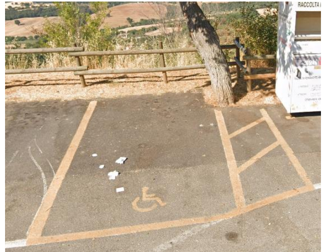
5 Reserved parking Via Foscolo
