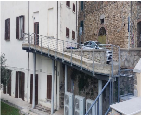
45 Rear Municipal Building and ramps
